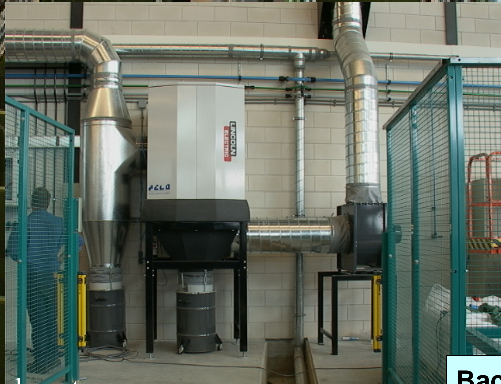
Central Fan controlled system
